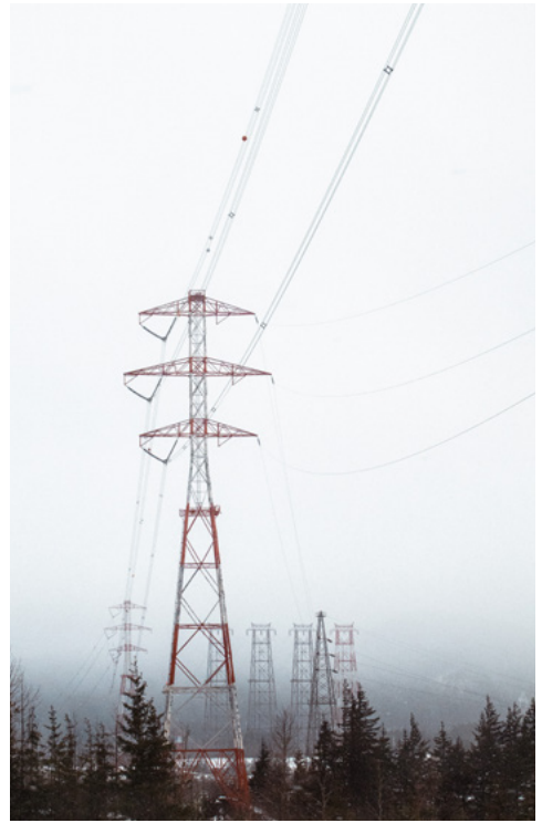
TRANSMISSION LINE TOWERS
